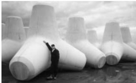
A tetrahedron ("four faces" in Greek) is a symmetric solid; such a solid has a crystal form and system of axes both called tetrahedral. The solid shown here, a gigantic concrete casting used to prevent erosion along the seacoast of Japan, has tetrahedral axes. Such a solid always stands upright no matter how it is dropped or turned.
